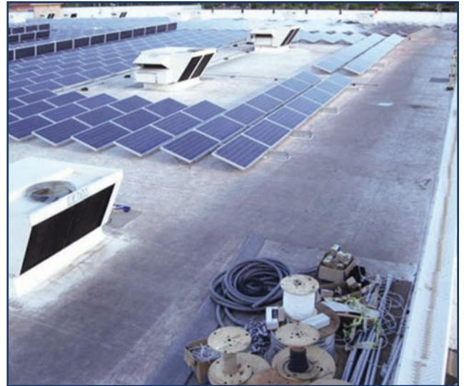
*Photo 1 – New TPO roof damaged during PV installation. Courtesy of Firestone Building Products.*
